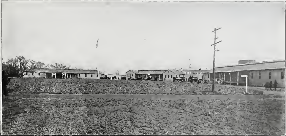
FIG. 117.—View of front of General Hospital No. 3.
